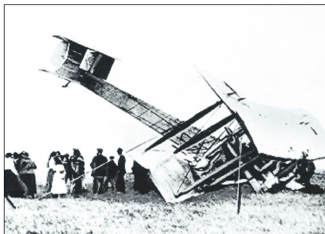
Alcock & Brown's landing in Derrygimlagh Bog, Ireland.
