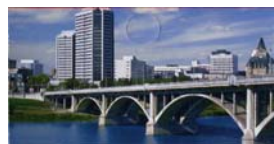
Broadway Bridge, Saskatoon, SK
